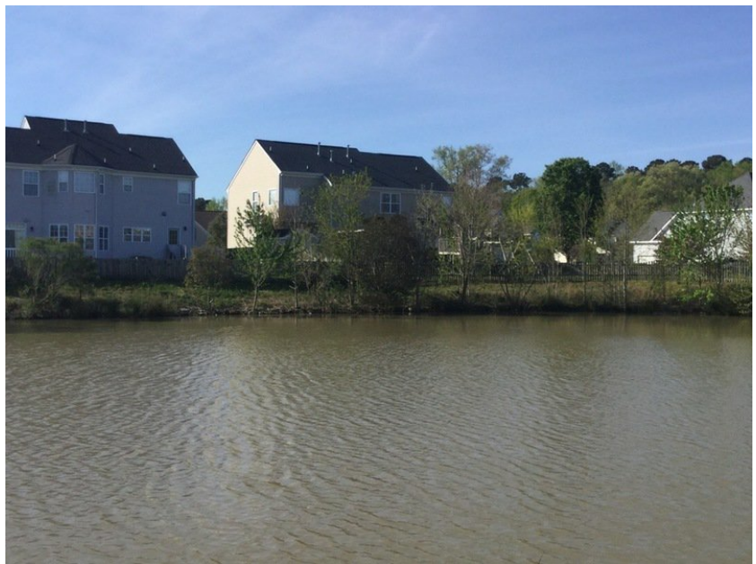
Trees and woody vegetation overgrown on slope around pond.
