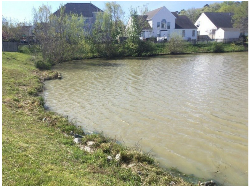
Grass filter strip cut too short along pond. It would seem to be in good condition if allowed to grow.
