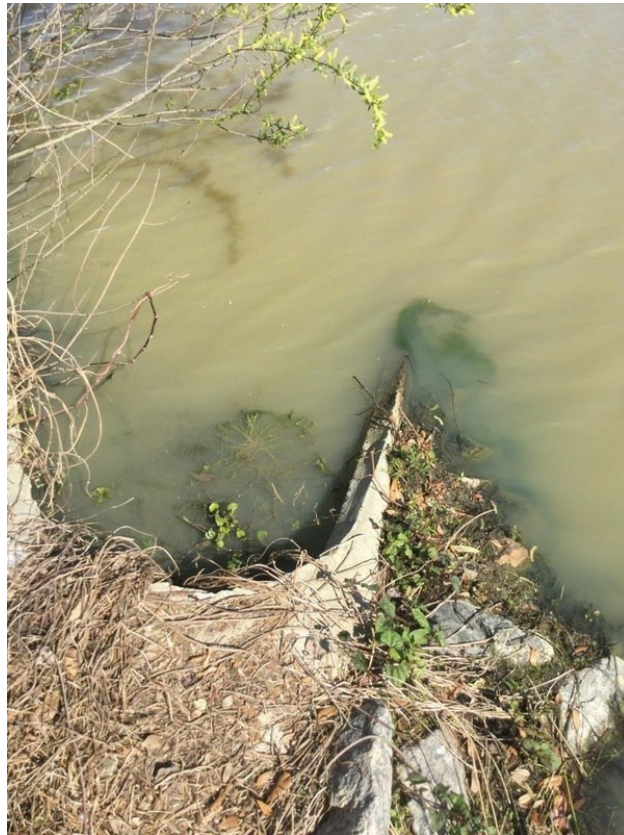
Aquatic vegetation growing inside of pipe. Also, woody vegetation growing around outside of pipe. Shown on map as a storm node.
