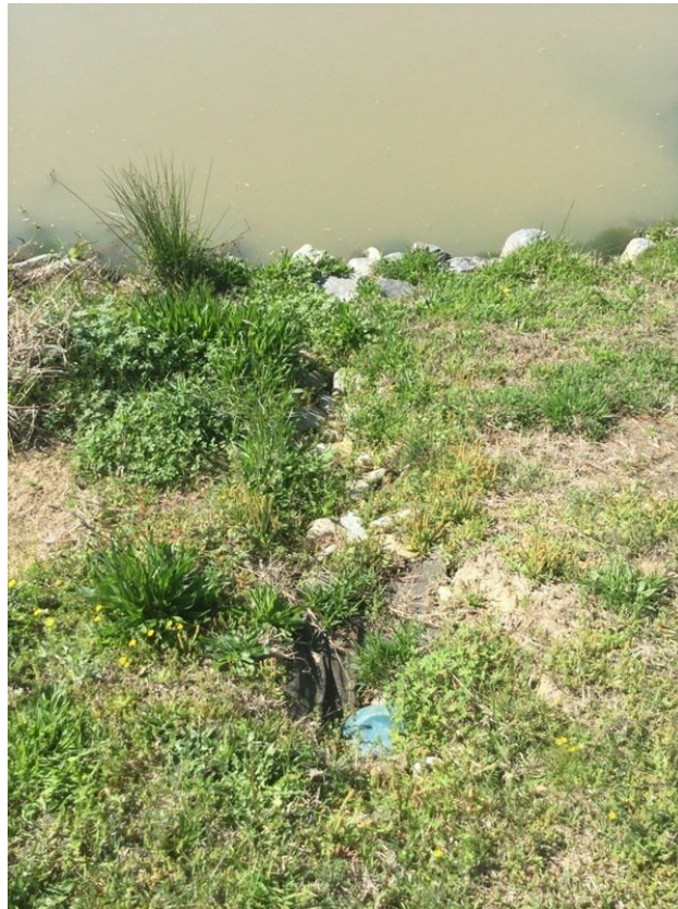
Structure built into slope. Possibly to drain private pool.
